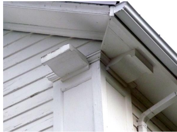
The crowning element on top of the pilaster on the First Baptist chapel at Crossroads (1836), reflecting the practice favoured by Smith in his wooden buildings of placing a modillion against the soffit.
