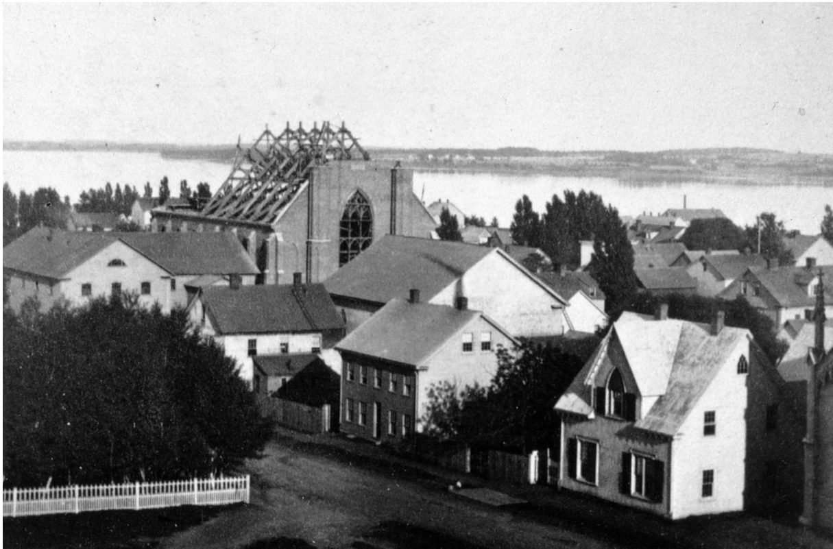
The new Wesleyan Chapel with more than half of the massive roof trusses erected that would create an unsupported span of almost seventy feet. The trusses were erected by Bertram Moore, who was, at the time, a citizen of Charlottetown and member of the church. 1863. PARO.
