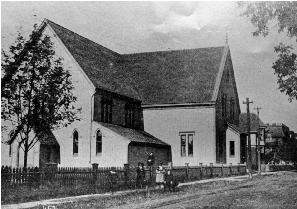
Photo of Upper Prince Methodist church (Grace Methodist) showing the 1884 lateral wing added to the 1877 building. c. 1890. PARO.
