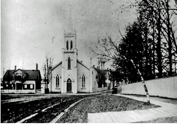
The Free Church of Scotland, on the northwest corner of Euston and Prince Streets, rented in 1871 to accommodate increasing congregations. PARO.
