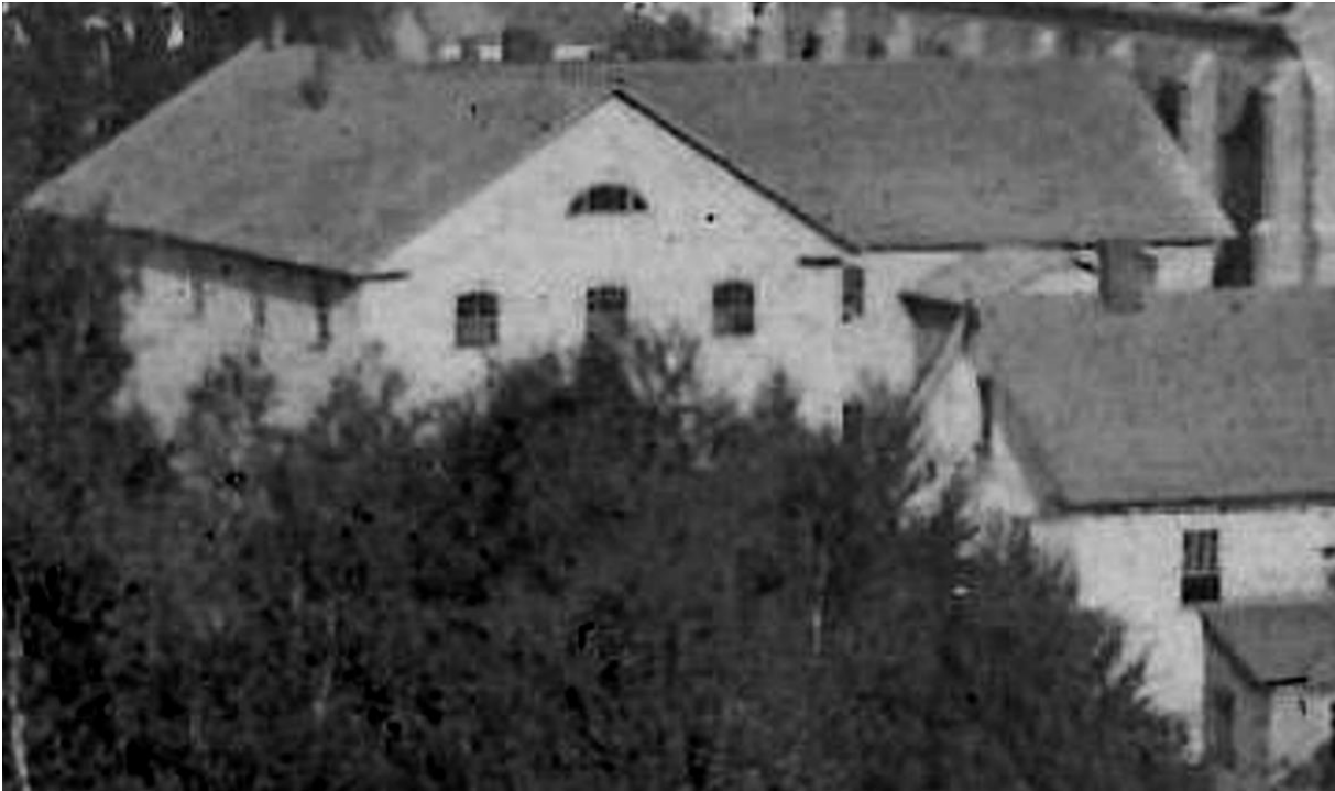
The 1835 Prince Street Methodist chapel after its enlargement in 1837 and further expansion at right angles in the middle of the south side of the first two phases of construction, in 1846, just eleven years after it was first built. Detail of 1863 photo, PARO.
